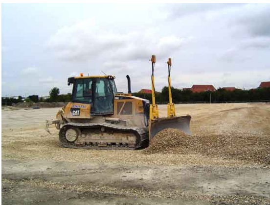
Laser-guided grading of a pitch
