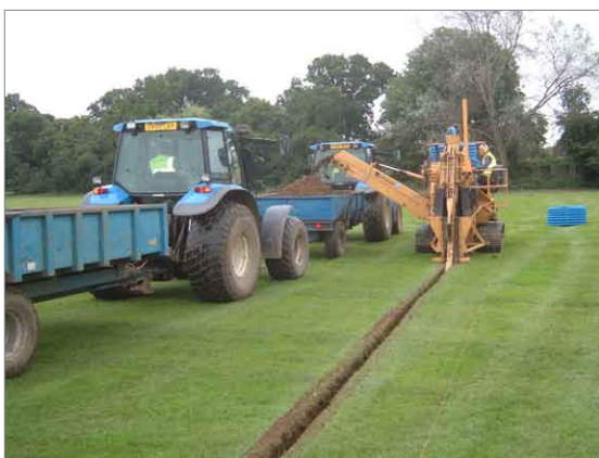
Drain installation normally requires the use of specialist trench machinery fitted with laser guidance
