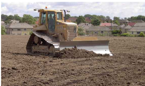
Many sites require major regrading of levels
